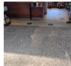
Source: Viracopos International Airport (VCP) - (Campinas / SP)
